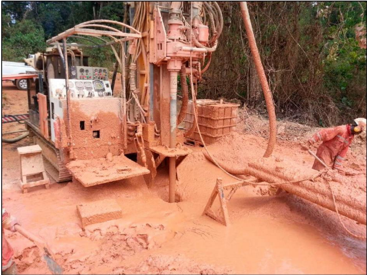
Figure 12 Diamond Drilling at KDW03 (after Golder, 2015a)
